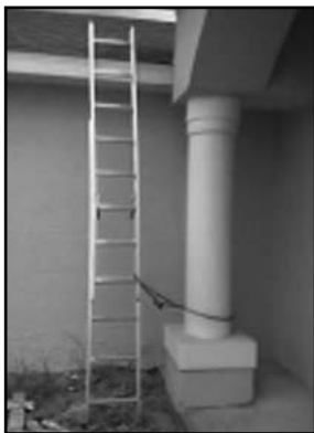
Example of target hardening of construction equipment.
