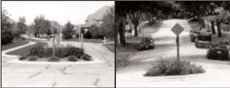
Traffic circles, of varying sizes, reduce speeds and crashes in residential areas.
