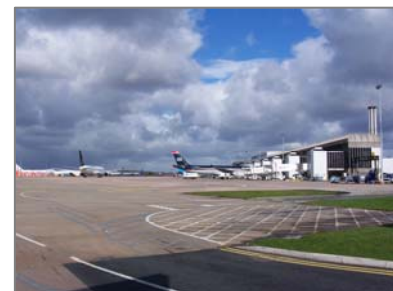
Manchester Airport (NW security gate, runway access and controlled runway area)
