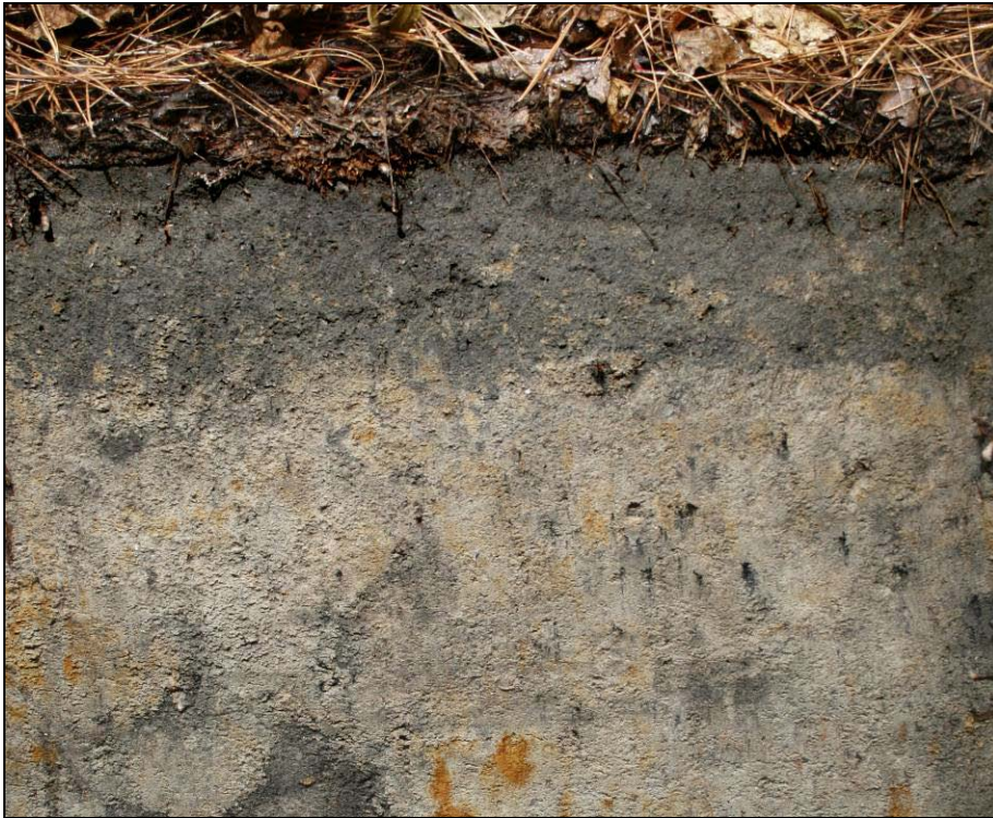
Figure 23. In this soil, a gleyed matrix begins immediately below the dark surface layer.
