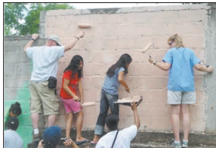
Every work project is a community effort.
