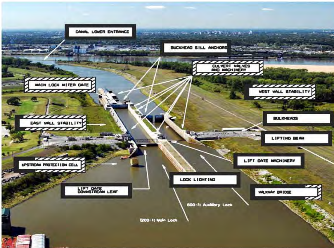
Aerial View of Lock No. 27 (Looking Downstream)
