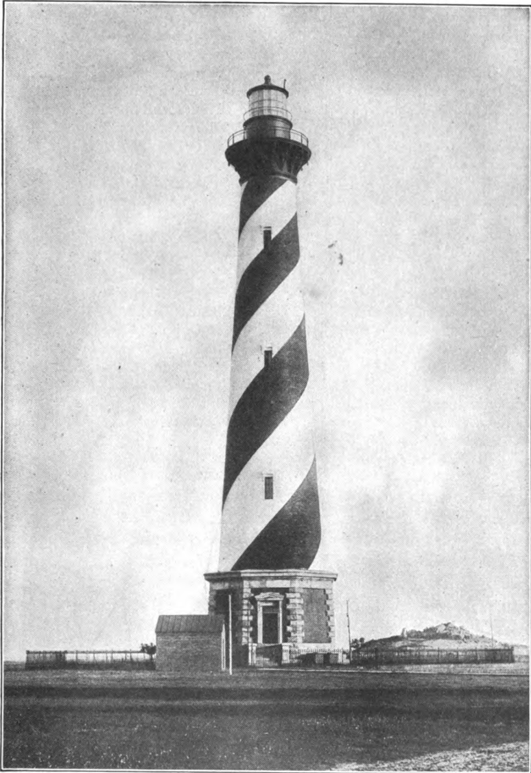
Cape Hatteras Light Station, N. C.
