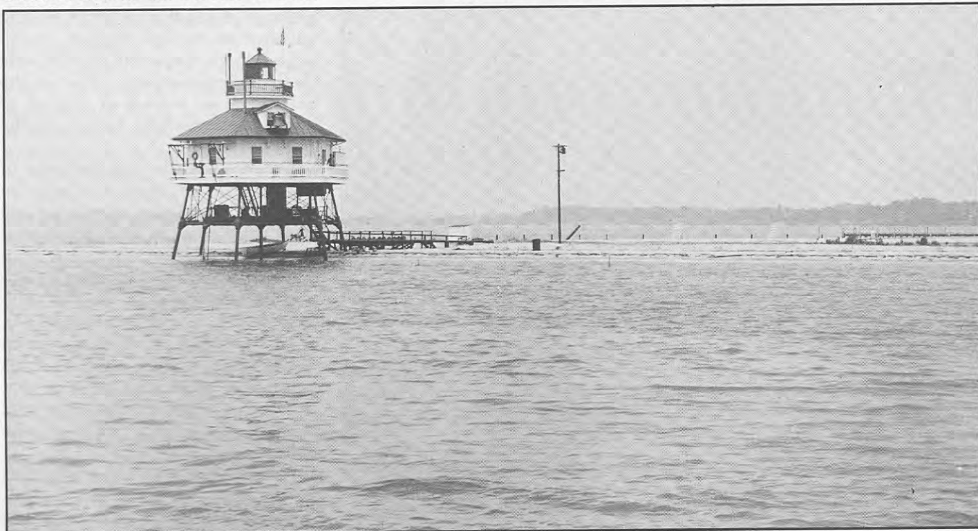
Drum Point Light, Maryland. This screw-pile light was saved from destruction and transferred to Calvert County Museum.
