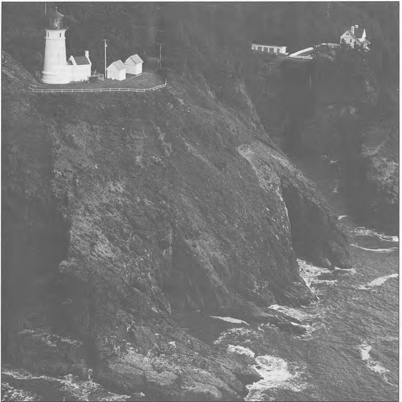
The building materials for the Heceta Head Lighthouse had to be landed from the tender and muscled up the cliff to the construction site. The photograph shows the high headlands typical of the topography of the Pacific Northwest.
