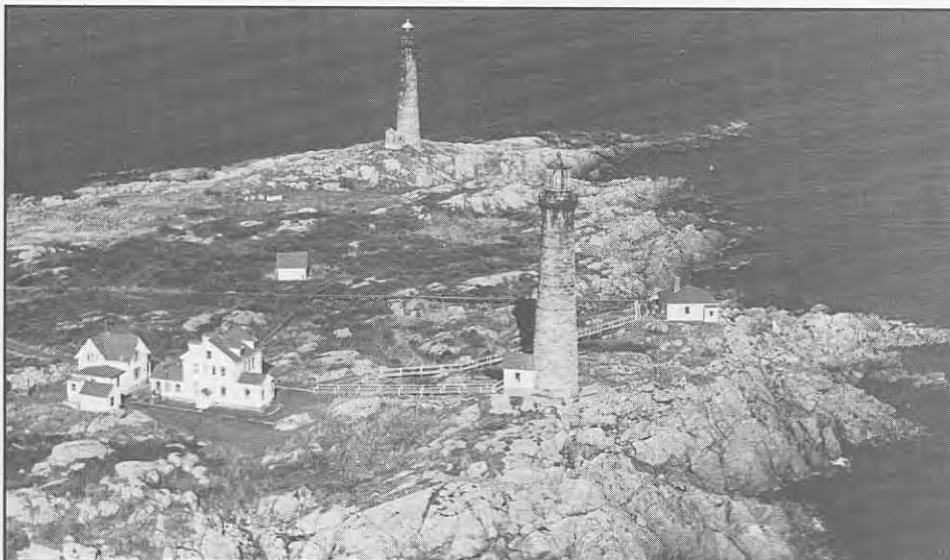
Twin tower lights, like these on Cape Ann, Mass., helped mariners determine which light they were seeing from a distance.
