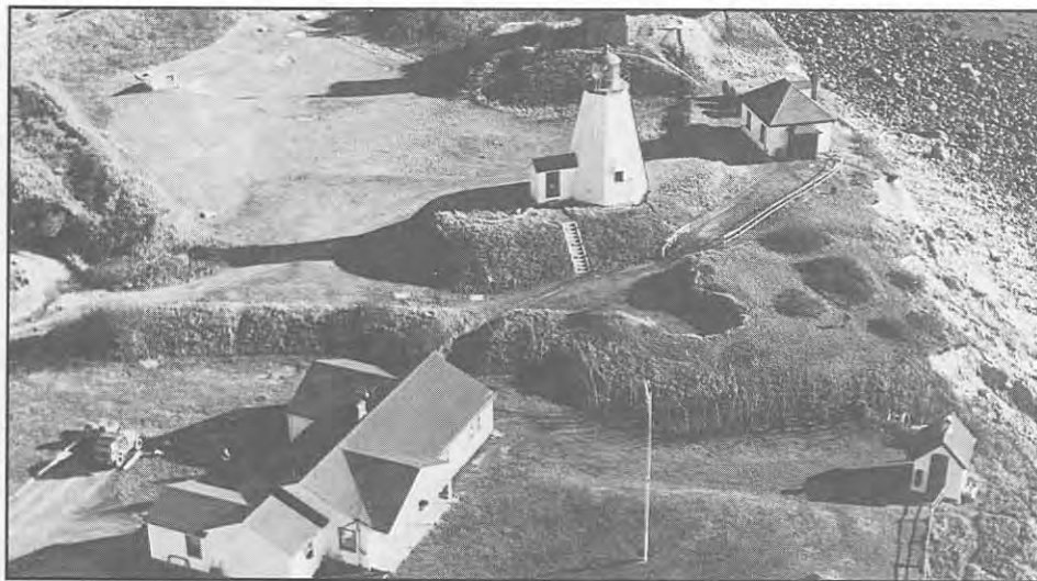
A light was first built on Gurnet Point, near Plymouth, Mass., in 1768. Hannah Thomas became America's first woman keeper when she relieved her husband. It was destroyed by fire and rebuilt as twin towers. The north tower was used until 1924. Notice the earthwork remains of the Revolutionary fort and the round base of the second tower.
