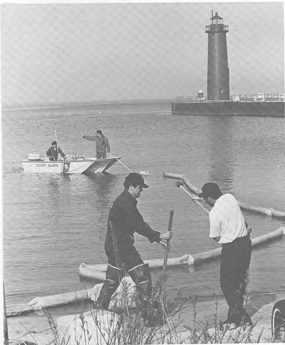
Response personnel deploy containment boom in Lake Michigan during Atlantic Strike Team/COTP Muskegon, Mich., drill.
