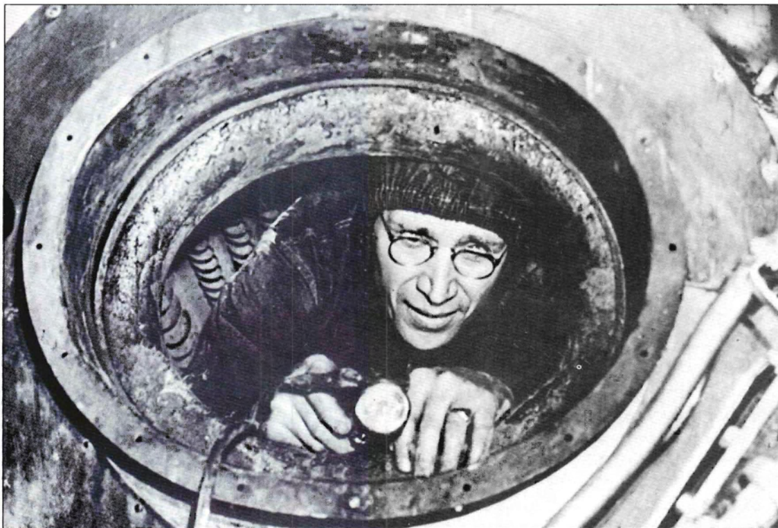
Left: A civilian marine inspector with the Bureau of Marine Inspection and Navigation climbs through a ship boiler during the 1930s. The inspectors periodically had to crawl through boilers and bilge compartments, looking for rust, loose rivets and wiggling valves.
