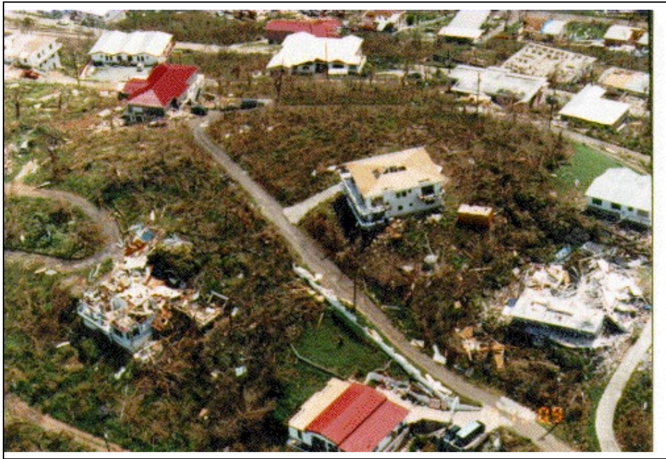
Figure 1-13. Residential damage on St. Thomas. (Photo courtesy of Brian Smith)
