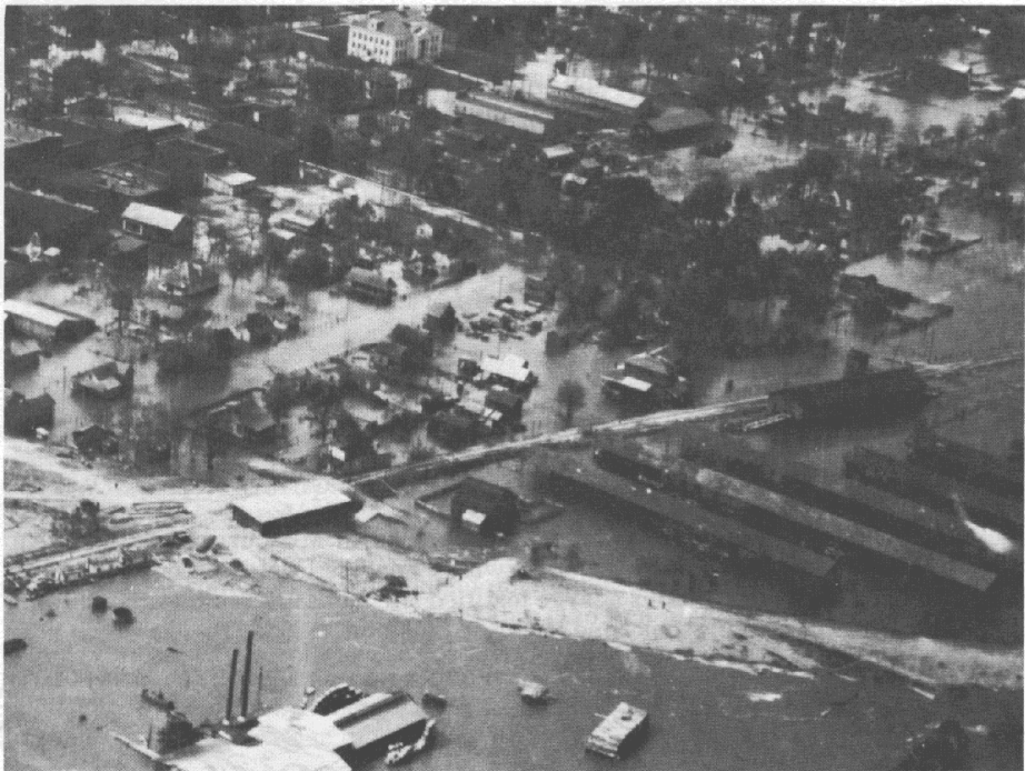
CREVASSE WATER. When the Dorena levee broke in 1927, water from the crevasse inundated the town of New Madrid, Missouri. In the above photograph, taken four days after the crevasse, the only completely dry land remaining in New Madrid is the levee in front of the town. It was reported a few days later that the water was higher in the town than it was in the Mississippi.
