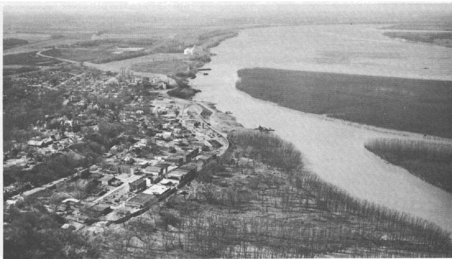
HICKMAN HARBOR. The Army Corps of Engineers completed a harbor project at Hickman, Kentucky, in 1963. The harbor now serves terminal facilities that handle grain, sand and gravel, and petroleum products. The industrial area includes about 130 acres. A floodwall and levee system to protect Hickman from flooding was also constructed by the Corps.
