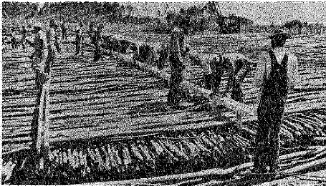
Bank protection—old style. Weaving of a giant willow mattress. (Photo by C. Fortier)
