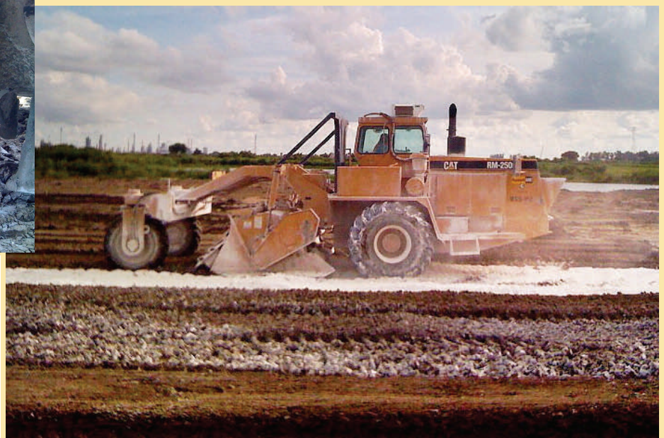
Working at the Bonnet Carre Spillway, a churner tractor (right) mixes lime with clay to provide a stabilized soil mixture that will be used at the EAM demonstration site on the Mississippi River Levee. Inset above: churner tractor "teeth" mix lime with the special clay.
