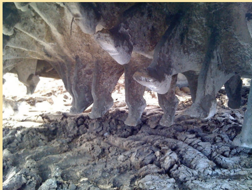
Working at the Bonnet Carre Spillway, a churner tractor (right) mixes lime with clay to provide a stabilized soil mixture that will be used at the EAM demonstration site on the Mississippi River Levee. Inset above: churner tractor "teeth" mix lime with the special clay.
