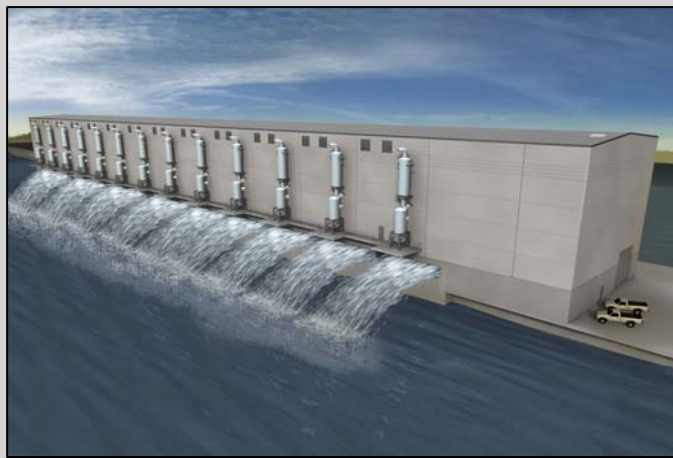
Above are conceptual illustrations of the West Closure Complex pump station. At left is the protected side, and at right is the GIWW side. (The illustrated pick-up trucks parked on the ramp provide scale.) (USACE Illustrations)
