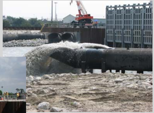
London Ave. Outfall Canal
