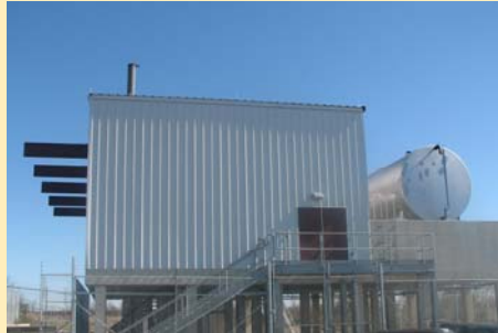
8 St. Bernard Parish Pump Stations
