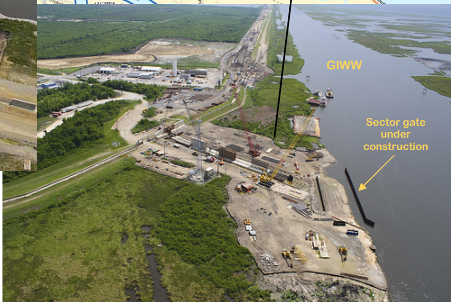
Above is a recent photo of the IHNC Surge Barrier being constructed across the MRGO and tying in to the new floodwall in St. Bernard Parish. At right is the on-going prep work for the IHNC Surge Barrier to tie-in to the levees on the north side of the GIWW .
