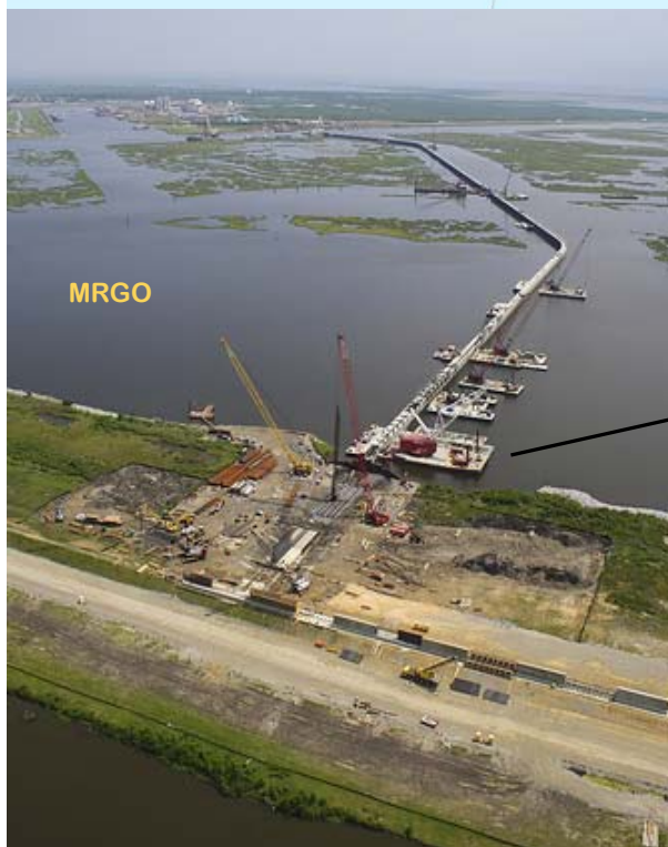
Above is a recent photo of the IHNC Surge Barrier being constructed across the MRGO and tying in to the new floodwall in St. Bernard Parish. At right is the on-going prep work for the IHNC Surge Barrier to tie-in to the levees on the north side of the GIWW .
