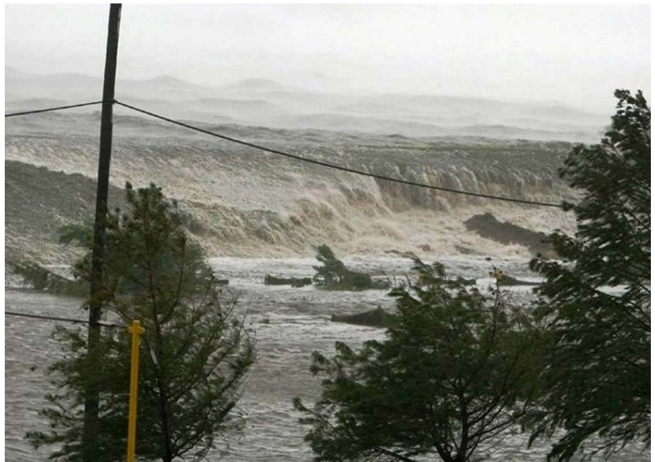
This dramatic photo shows Hurricane Katrina’s surge overtopping levees under the Paris Road Bridge adjacent to the Entergy power plant in New Orleans East.
