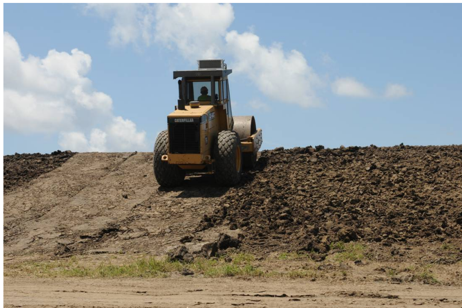
A tractor-pulled steel drum roller (above) and self-propelled steel drum roller (below) make parallel and perpendicular passes on a levee. A steel roller compacts and "seals" the surface of an under-construction levee. (USACE Photos)
