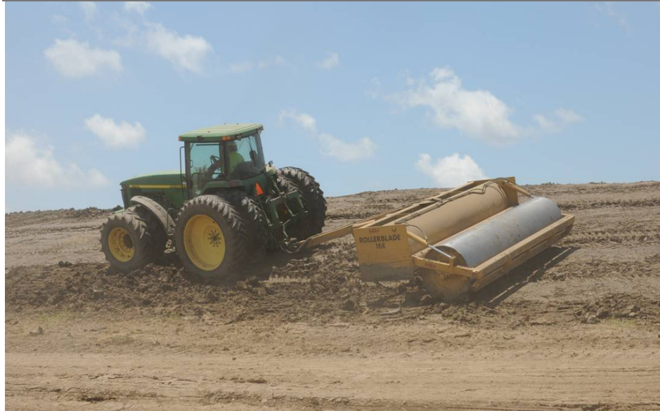
A tractor-pulled steel drum roller (above) and self-propelled steel drum roller (below) make parallel and perpendicular passes on a levee. A steel roller compacts and "seals" the surface of an under-construction levee. (USACE Photos)
