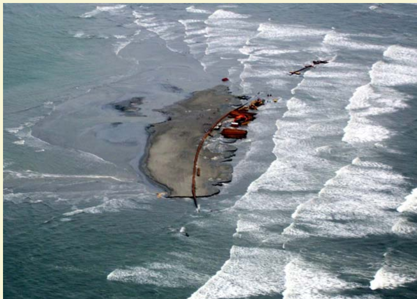
Reach E-4 of the sand berm at the Chandeleur Islands
