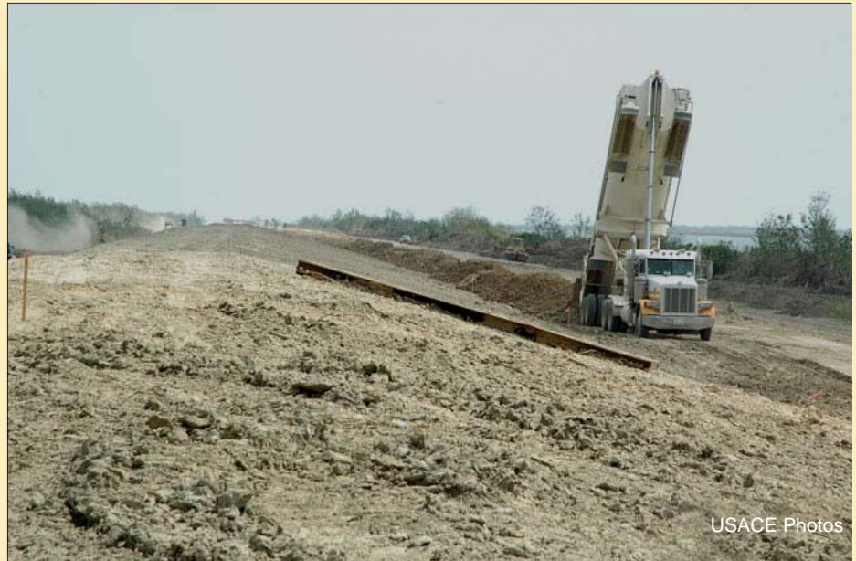
A dump truck empties its load of approved clay at a levee-building site.
