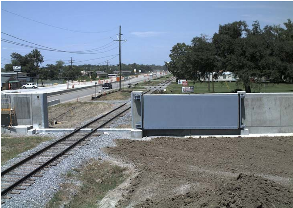
The railroad gate along Highway 23 in St. Bernard Parish will be closed to prevent storm surge prior to a tropical event. USACE Photo by Tom Durel
