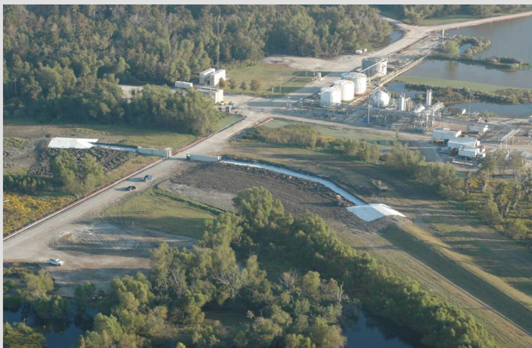
Almedia Drainage Structure
