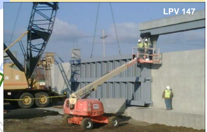
LPV 147 Last month, the Hwy. 46 north and south gates were installed across the roadway. These are the largest highway gates in the system.
