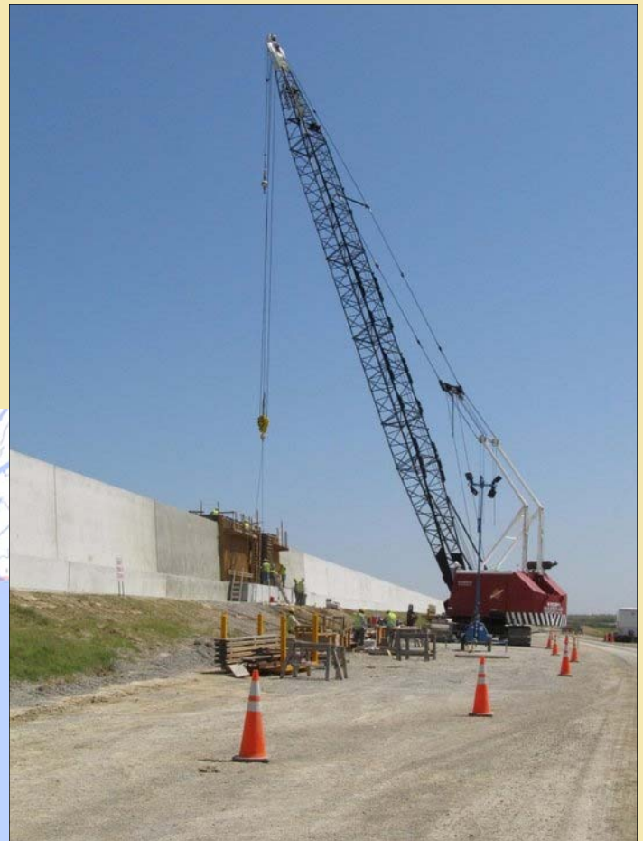
Above: Workers install the last monolith in the LPV 145 floodwall on March 21. This occasion marked the achievement of 100-year designation for that stretch of the St. Bernard floodwall. Below: The completed floodwall section
