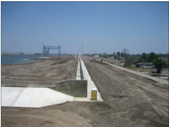
ABOVE: IHNC floodwall at Lower Ninth Ward just after construction.
