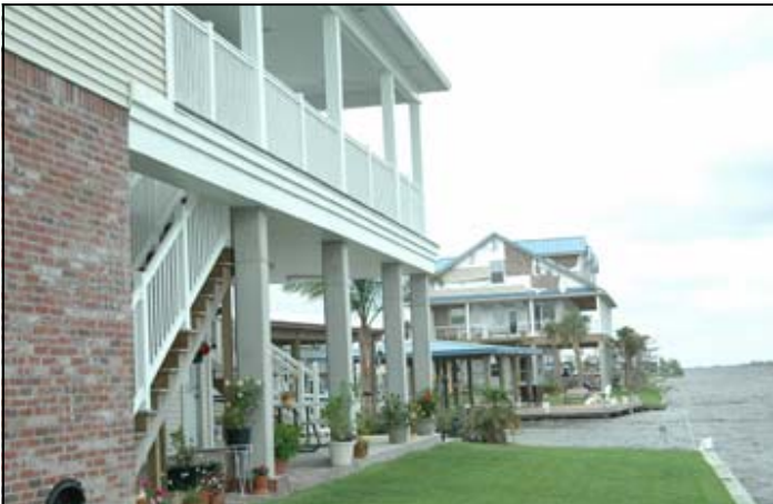
This is another example of a “non-structural” feature.
