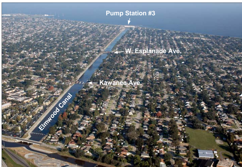
The SELA program enlarged and added concrete lining to the entire length of the Elmwood Canal, and recently completed improvements to Pump Station #3. SELA projects also include the bridges at Kawanee Ave. and W. Esplanade Ave. (USACE photo by Scott Riecke)
