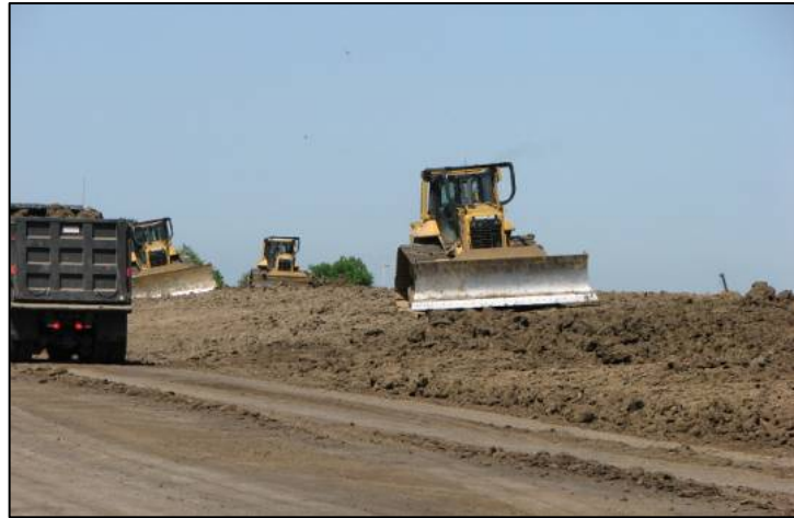
Verret to Caernarvon levee work
