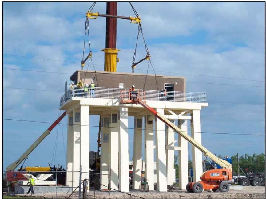
Lake Cataouatche Pump Station Safe House
