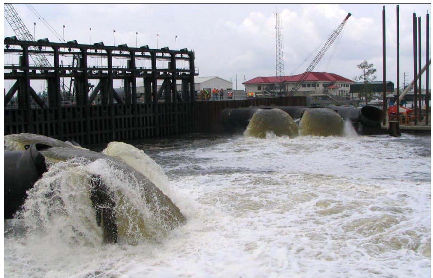
17th Street Canal pumping demonstration
