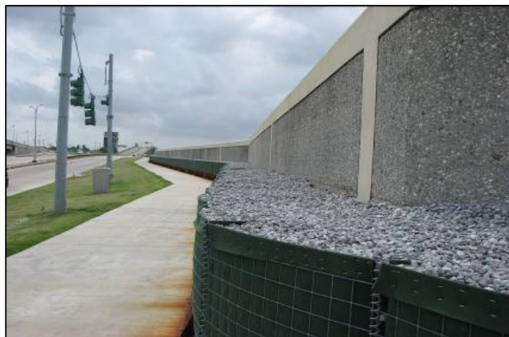
New Orleans Lakefront floodwall stabilization
