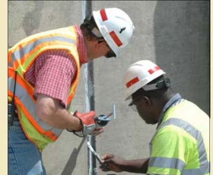
At left, construction workers remove expansion joint material from floodwall joint. Top, after placing Corps-approved material in floodwall joint, workers replace sealer.
