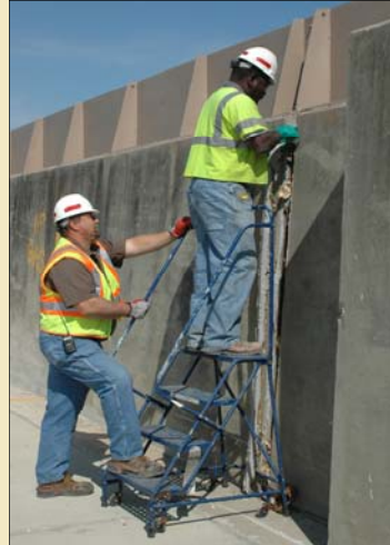
At left, construction workers remove expansion joint material from floodwall joint. Top, after placing Corps-approved material in floodwall joint, workers replace sealer.
