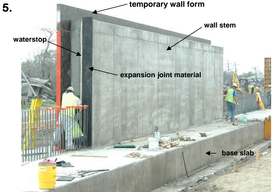
Typical Floodwall Expansion Joint
