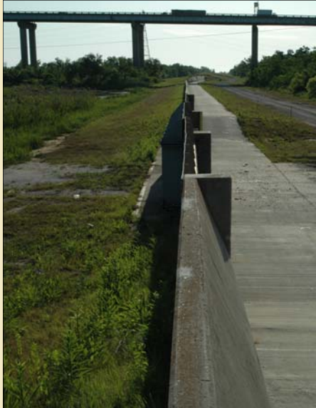
Paris Road bridge floodwall
