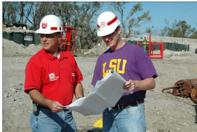
Engineers from the U.S. Army Corps of Engineers review plans at the London Avenue Outfall Canal during a regular check of on-site construction work. USACE Photo)
