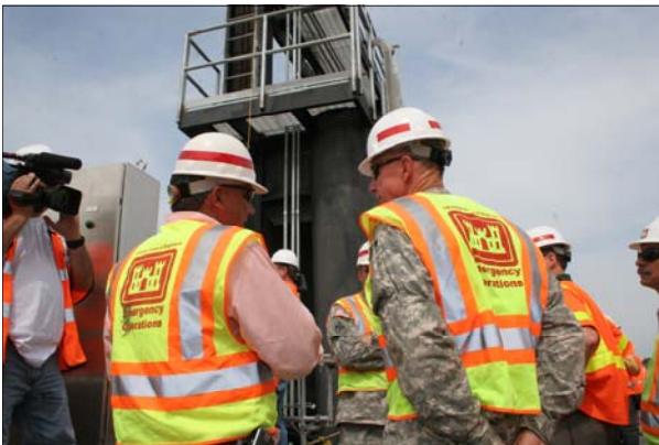
Senior Project Manager Jim St. Germain, left, gives the Chief a tour of the 17th Street Canal pumps and gates.
