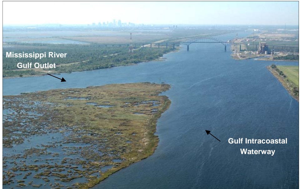
This aerial photo shows the confluence of the Gulf Intracoastal Waterway (GIWW) and the Mississippi River Gulf Outlet (MRGO), the general location of the Corps' proposed surge protection project. (USACE Photo)
