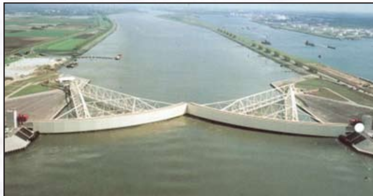
(Below) The Maeslant Barrier structure in the Netherlands automatically closes when needed. It is the largest moving structure on earth. A storm event on Nov. 8, 2007 closed the structure for the first time since being completed in 1997.
