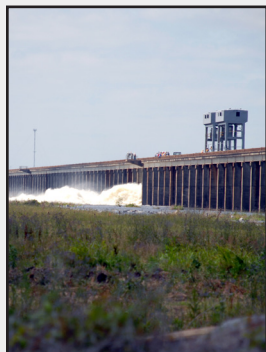
On the Cover: On May 14, 2011, the Corps operated the Morganza Floodway Control Structure for only the second time. Repairing the damage that occurred during use is a top priority for the New Orleans District. Photograph by Jenny Marc.
