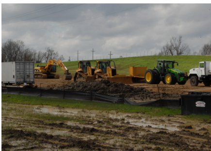
Left: Crews are constructing a seepage berm adjacent to the Mississippi River levee at Duncan Point in Baton Rouge, La. This project was ranked as the highest MR&T priority area in the New Orleans District's area of responsibility (photograph by Lee Mueller).
