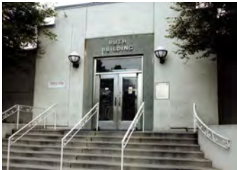
Facilities in Bethesda, Md., served as agency headquarters from 1996 to 2011. Buildings included the Ruth Building, at left, opened June 15, 1942, as part of the Army Map Service and named for Army Capt. Charles H. Ruth, first commanding officer of the Army Engineer Reproduction Plant
