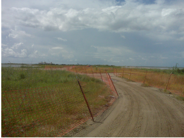
Safety fence is used to minimize impacts on the access trail.
