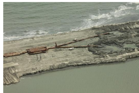
E4 North Berm Construction – August 26, 2010
