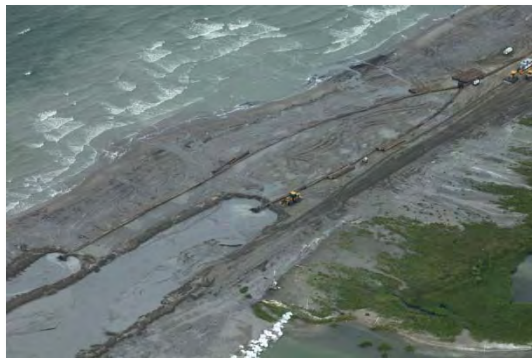
W9 Berm Construction – August 5, 2010
