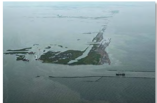
W9 Berm – August 5, 2010
