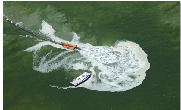
E4 Berm 6A refill – July 27, 2010
