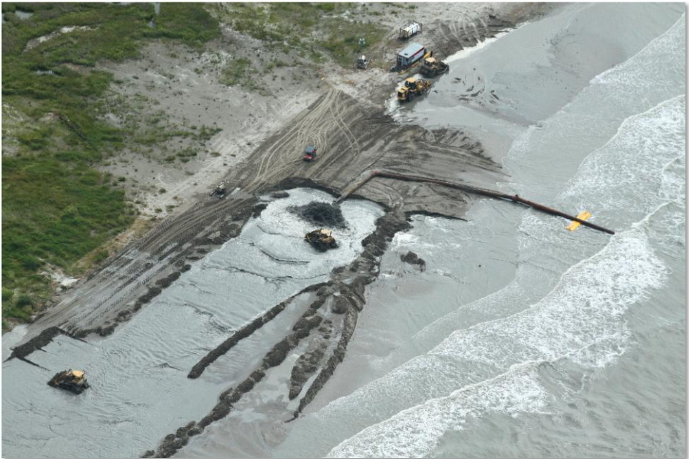
W9 Berm Construction – July 27 th , 2010
