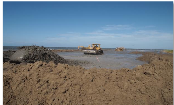
W9 Berm Construction – July 27, 2010
