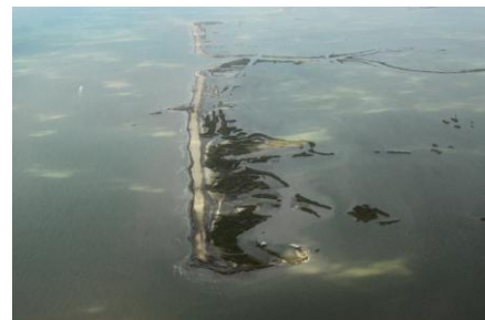
W10 Berm – November 28, 2010
