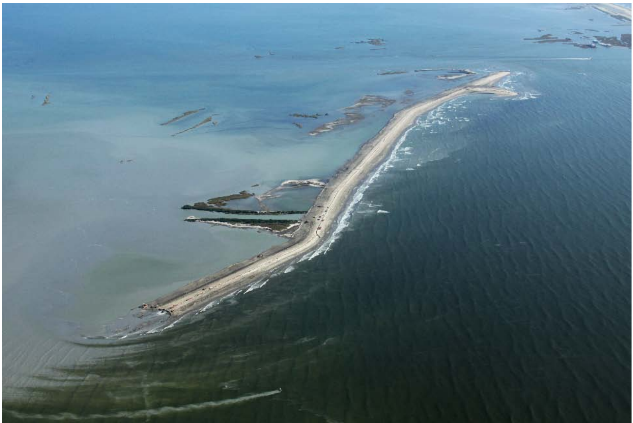
W8 Berm Operations – November 23, 2010
