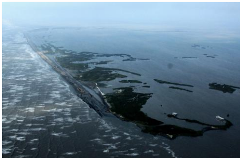
W10 Berm – November 16, 2010
