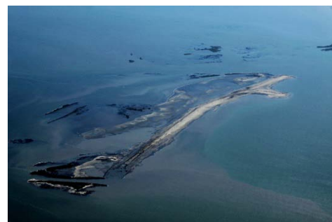
W8 Berm – November 7, 2010
