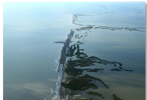
W10 Berm – November 3, 2010
