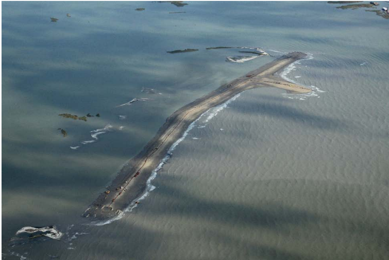
W8 Berm – November 3, 2010
