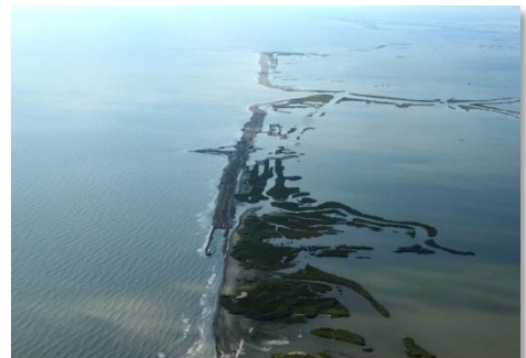
W10 Berm – November 3, 2010
