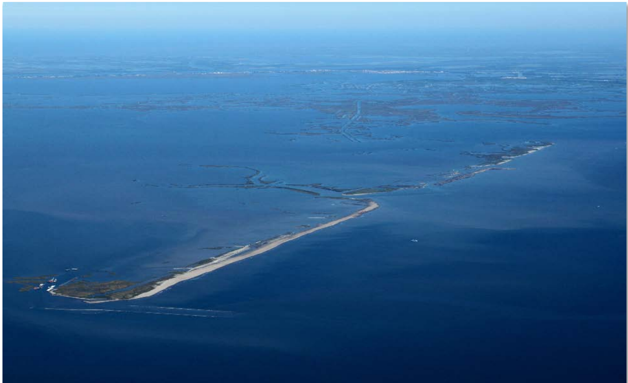
W9 & W10 Berm – October 7, 2010
