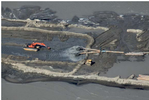
W10 Berm Operations – October 6, 2010
