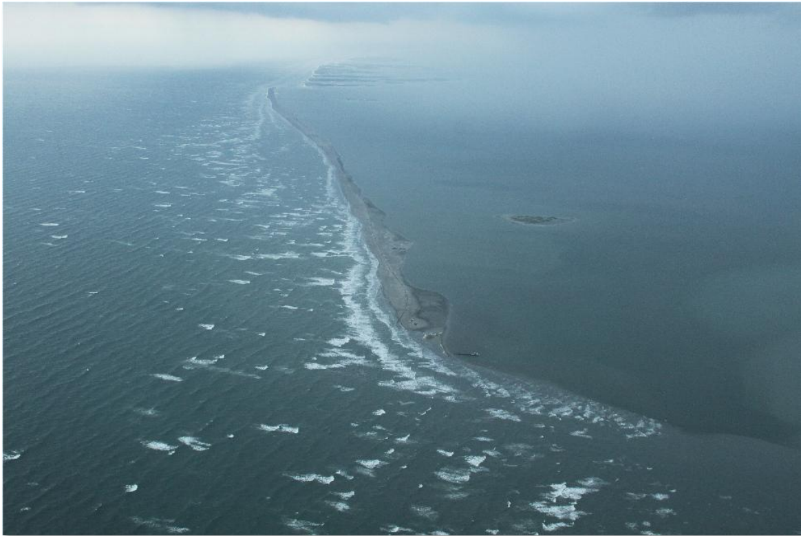
E4 North Berm – September 23, 2010
