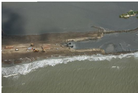
W9 Berm Operations – September 23, 2010
