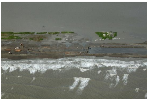
W9 Berm Operations – September 13, 2010
