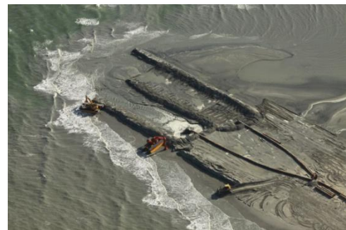
E4 North Berm – September 13, 2010
